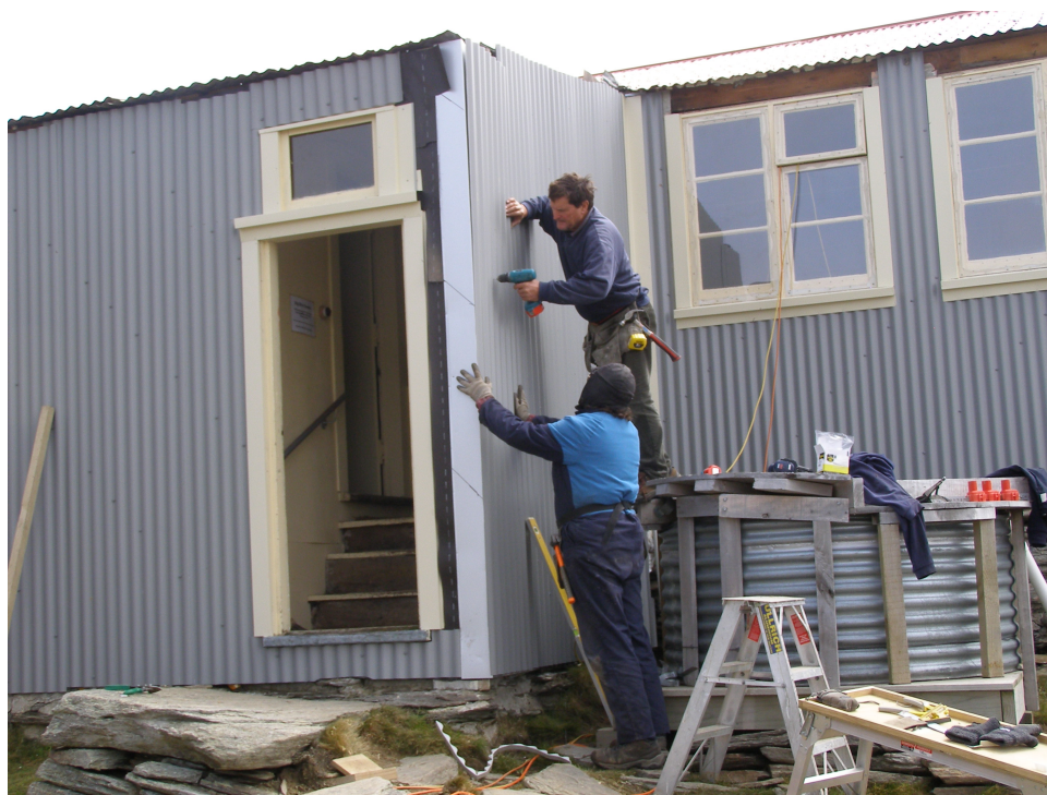
Being battle prepared: newly colour steel armoured. Geoff and Peter at work. KDM
