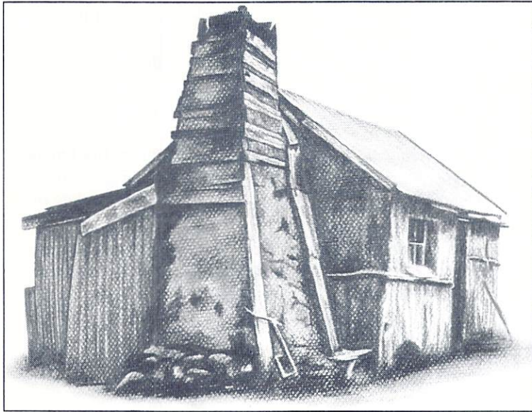
At the time of Tucket's historic journey there were a handful of European houses in the Otago Harbour region, mostly made from mapou logs and battens plastered in a clay and grass mixture.
